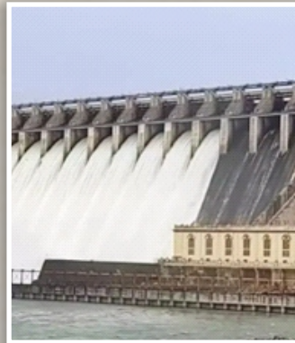
NAGARJUNA SAGAR DAM, KRISHNA RIVER
