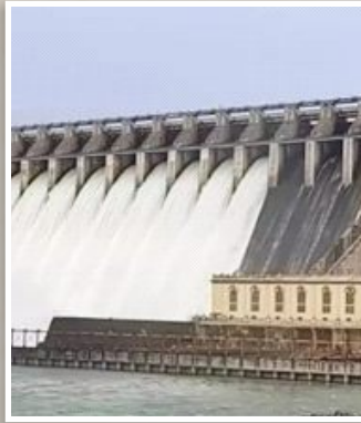
NAGARJUNA SAGAR DAM, KRISHNA RIVER
